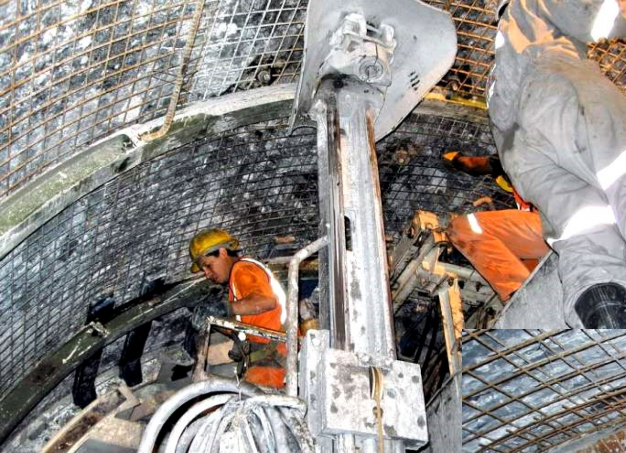
Original Olmos support system – wire mesh under steel sets installed inside finger shield
