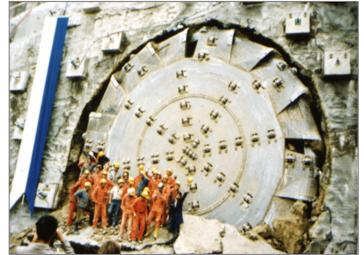
Following that success, the size of TBMs grew steadily also for application in more or less cohesive soils. Part of the Grauholz tunnel in Switzerland had to be driven through glacial deposits with an 11,80 m Slurry-TBM, which had been converted into an open face TBM for the stretch through stable marls.
