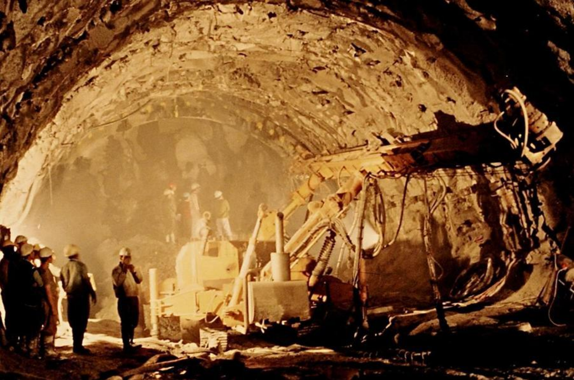
Forepole installation in the Daj Khad fault zone
