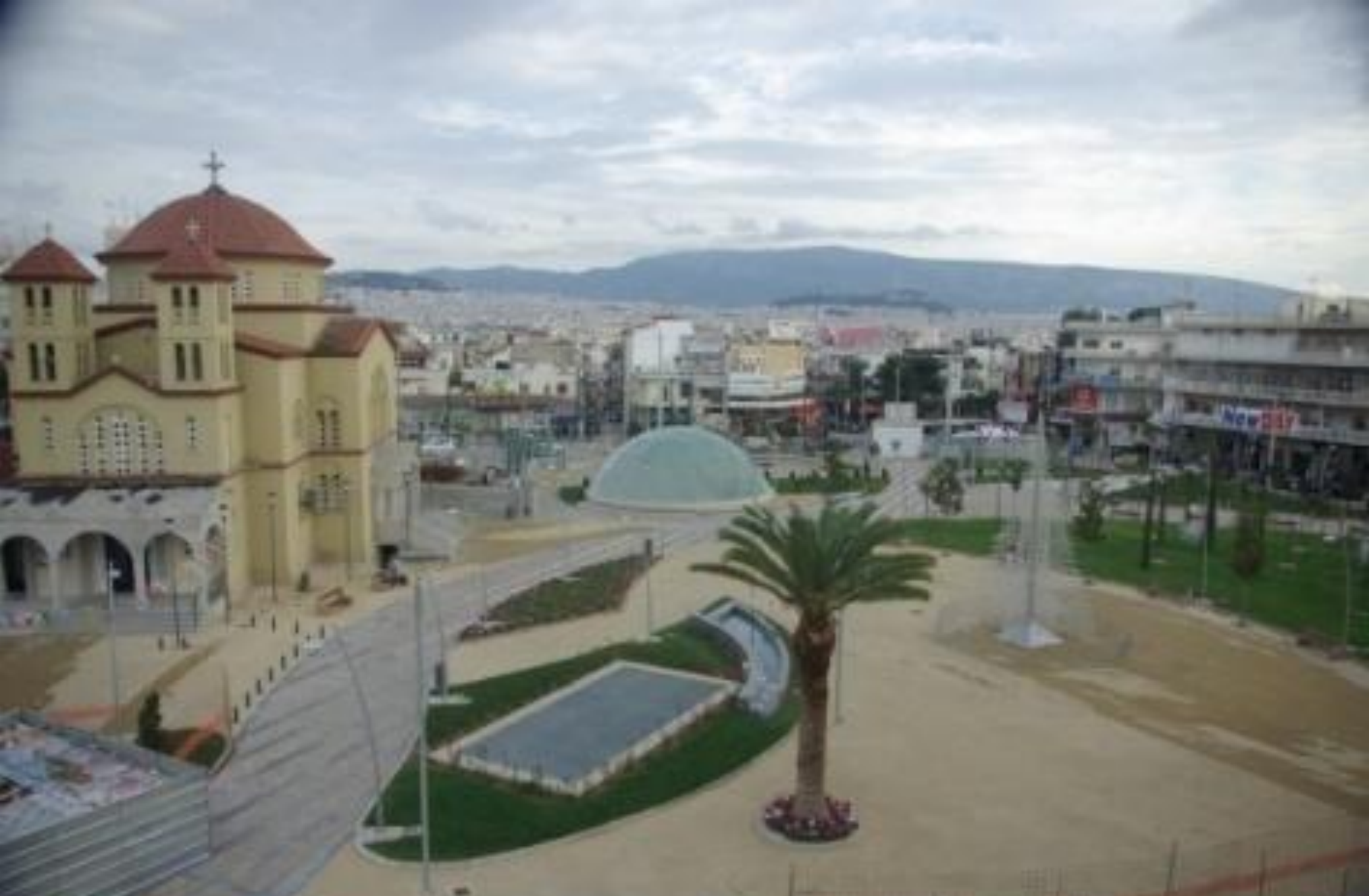
Peristeri Station – street level – during reinstatement – natural light dome
