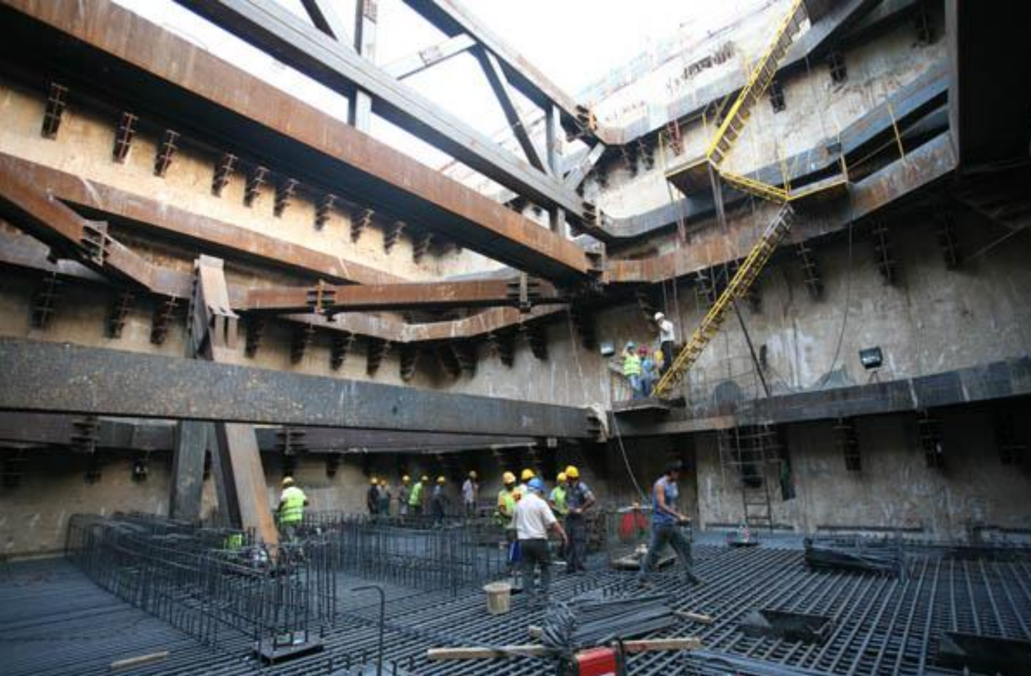
Station construction works – Temporary supporting struts
