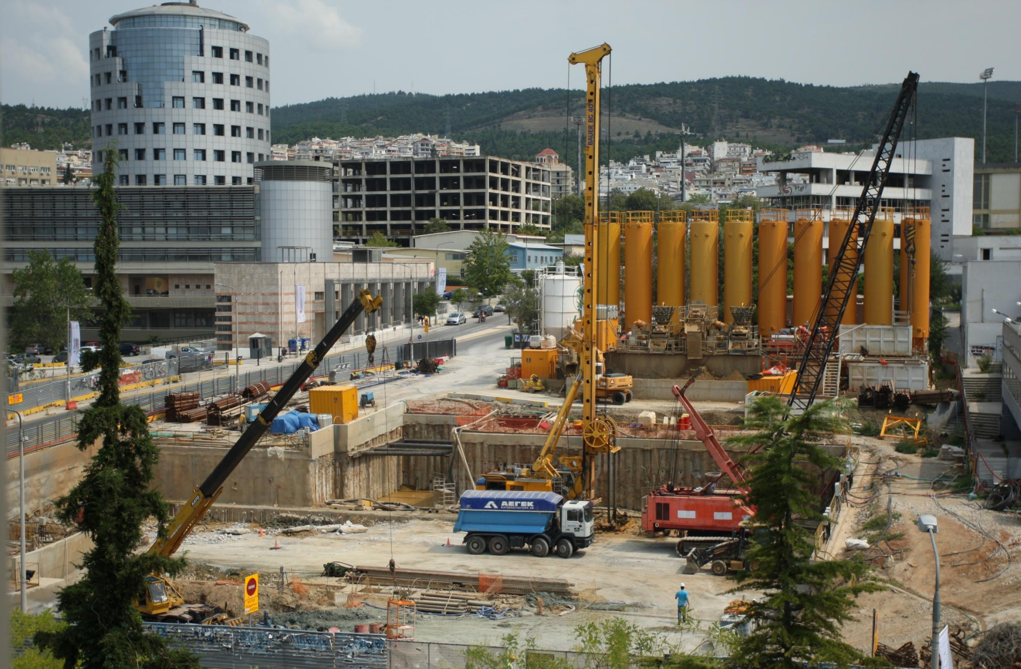
Diaphragm walls construction for Panepistimio station - Thessaloniki
