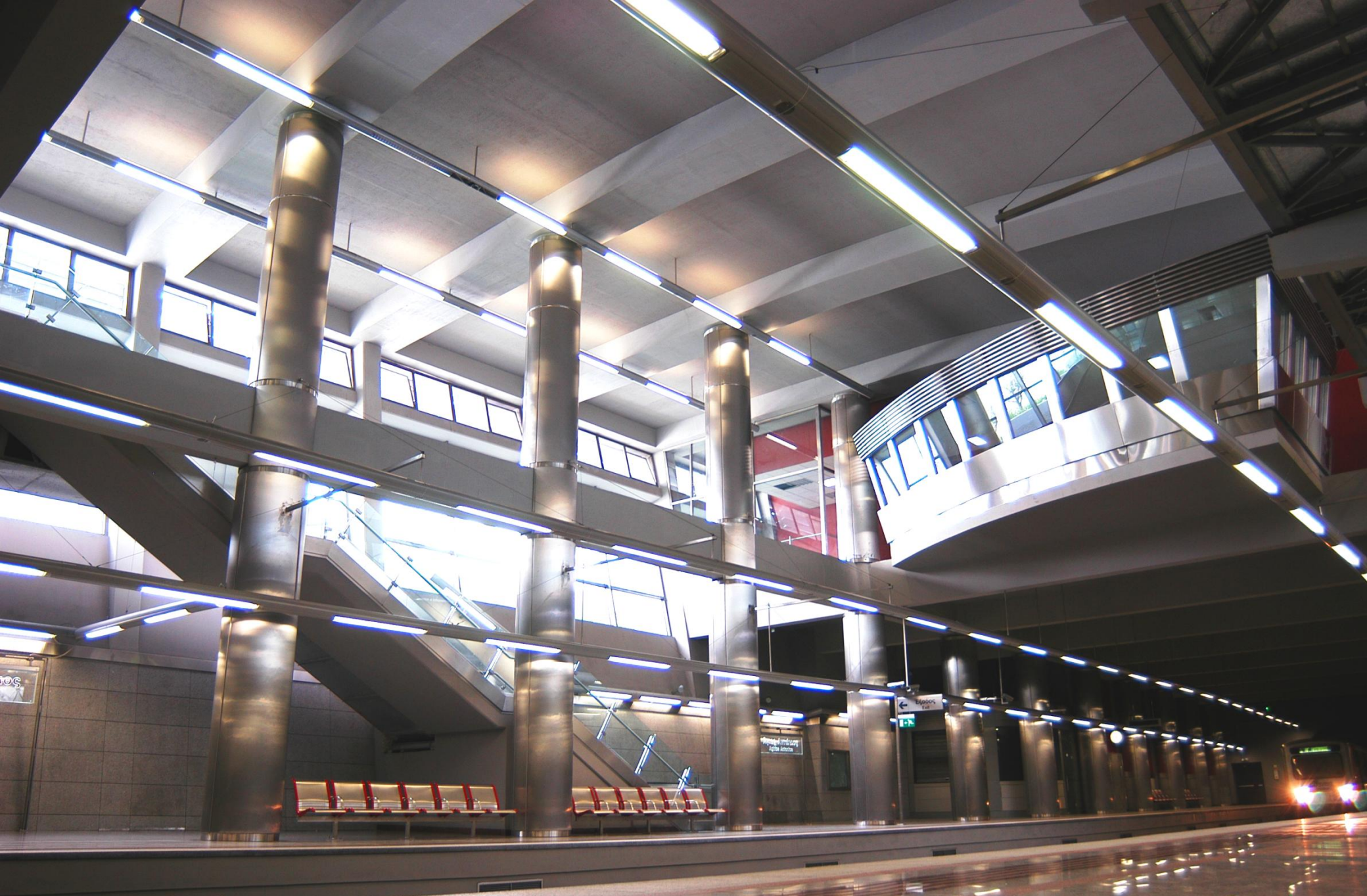
Agios Antonios Station – platform level – open architecture – natural lighting
