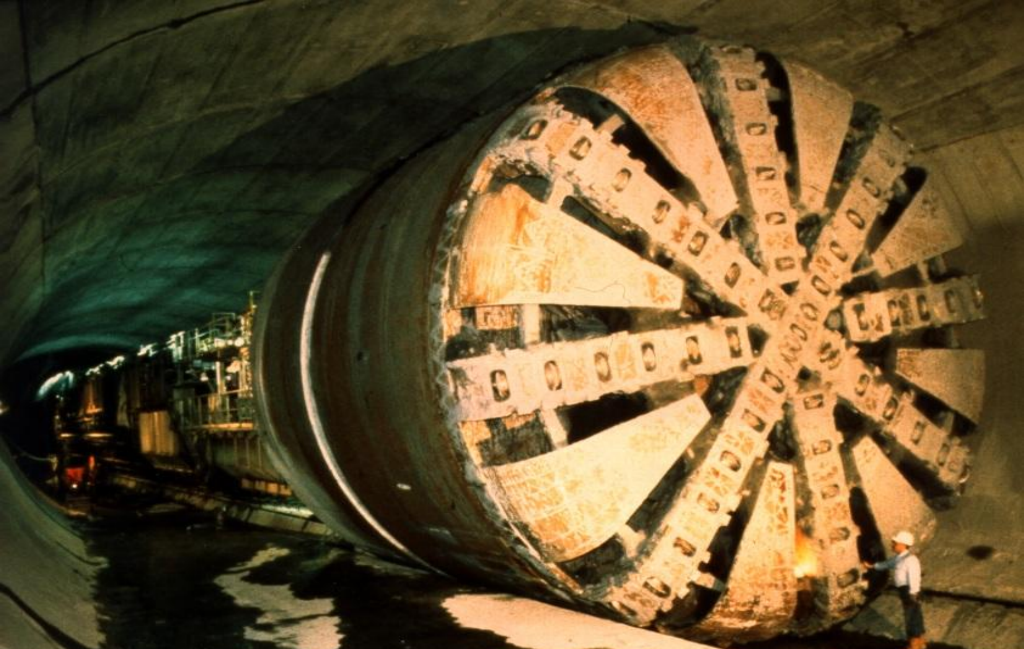
TBM – moved through the platform level of an NATM station
