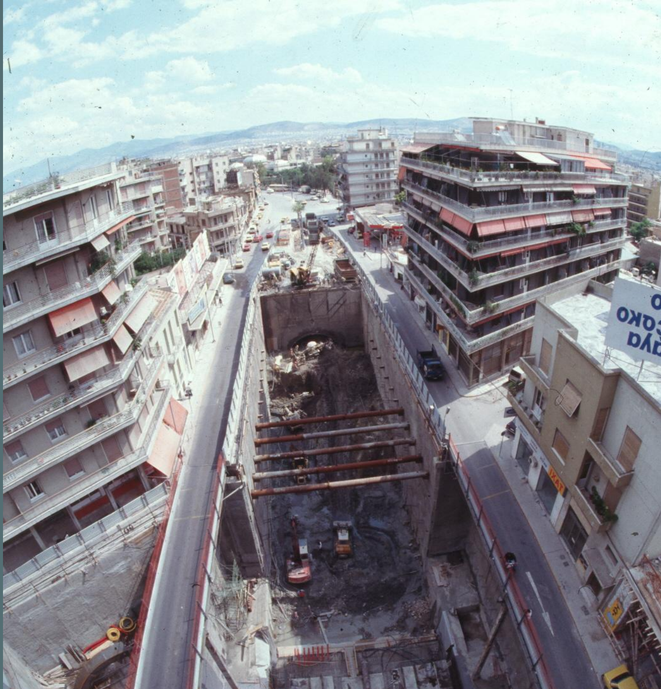
Cut and Cover – Neos Kosmos station, between buildings
