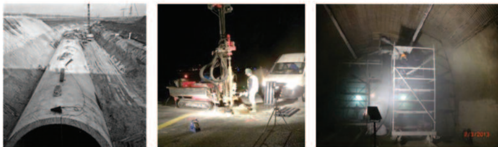
Figure 1. Worksite views: construction worksite (1974), geotechnical survey (2011) and strengthening worksite (2013)
