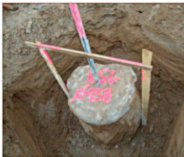
Figure: Jet Grouting excavated column
