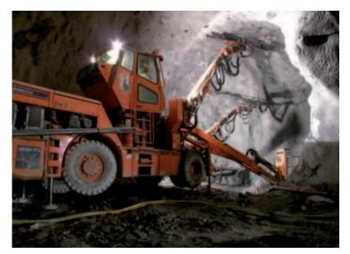
Fig. 1: Conventional tunnelling by drill an blast
