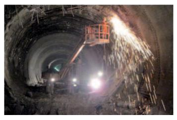
Fig. 3: Tunnel reconstruction due to unexpected high convergences
