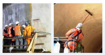
Figure 10 : Example of integrity testing to detect and repair pinholes, voids and other defects in membranes
