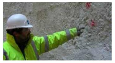
Figure 5: Quality assurance of sprayed membranes: visual identification of defects
