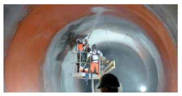
Figure 7: Two colour application of waterproofing membrane (1st coat orange, 2nd coat white)
