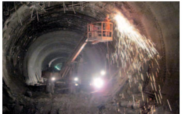
Fig. 3: Tunnel reconstruction due to unexpected high convergences
