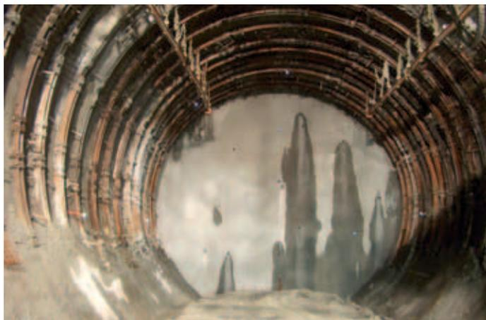
Fig. 4: Conventional tunnel drive (full face excavation by drill and blast, support with steel ribs, spiles, shotcrete and rock bolts)
