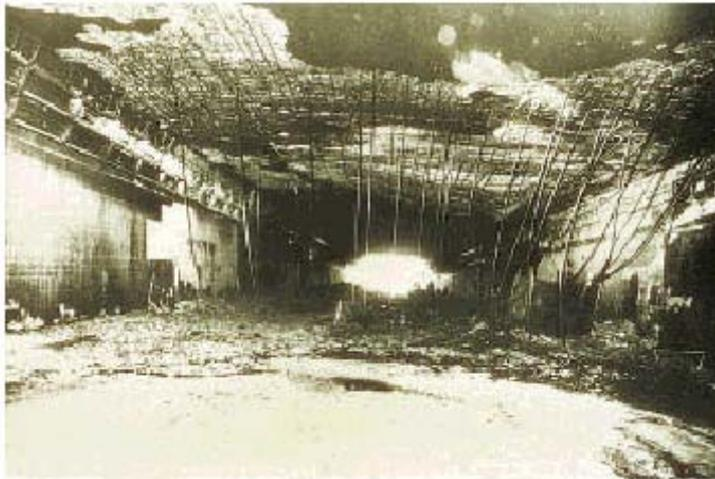
Figure 1: Completely destroyed pre-stressed concrete roof following a lorry fire in the Moorfleet/Hamburg motorway tunnel in 1968
