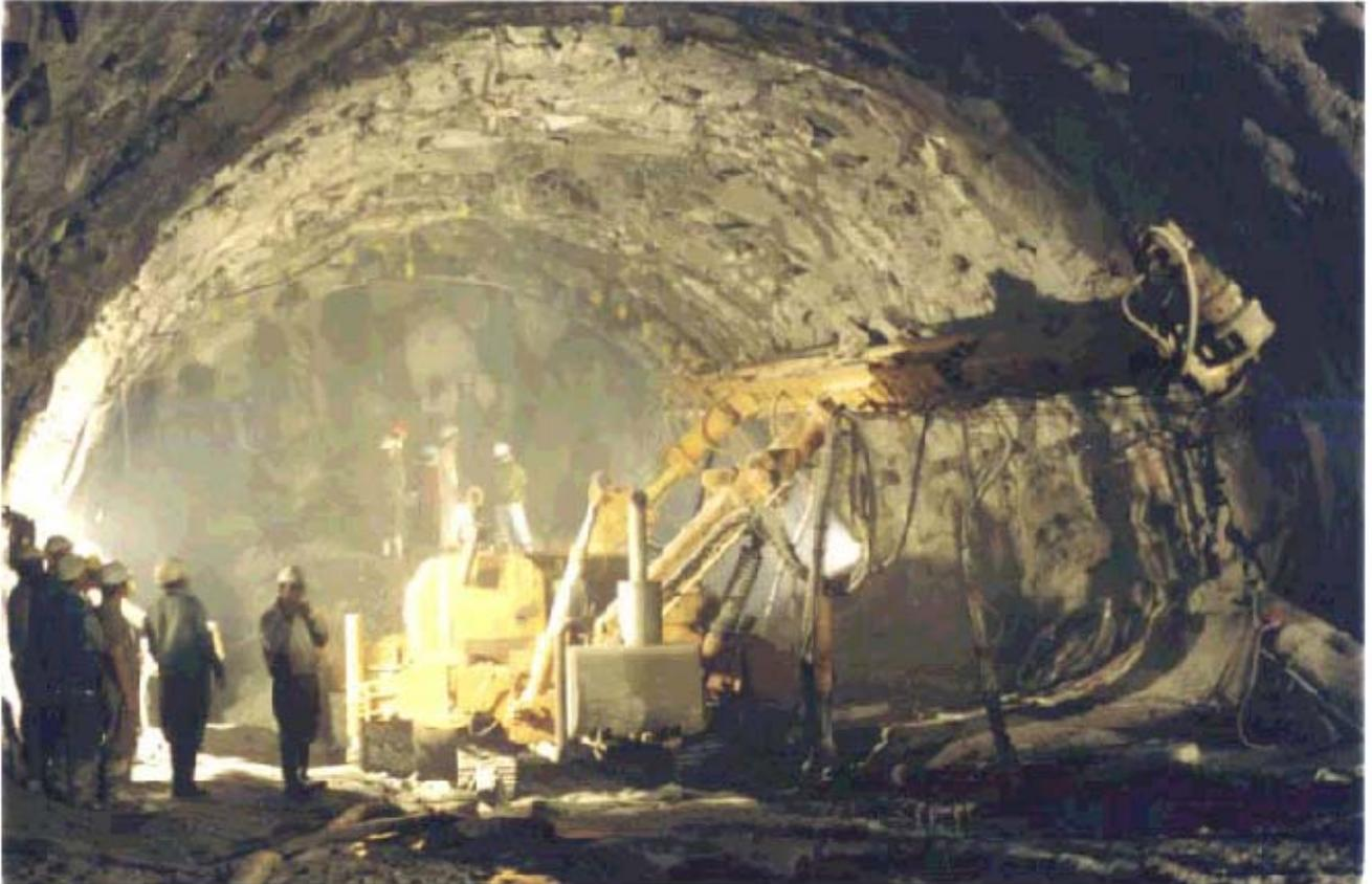
Figure 12: Installation of 12 m long grouted pipe forepoles to form a protective reinforced rock umbrella under which excavation of the top heading can proceed.
