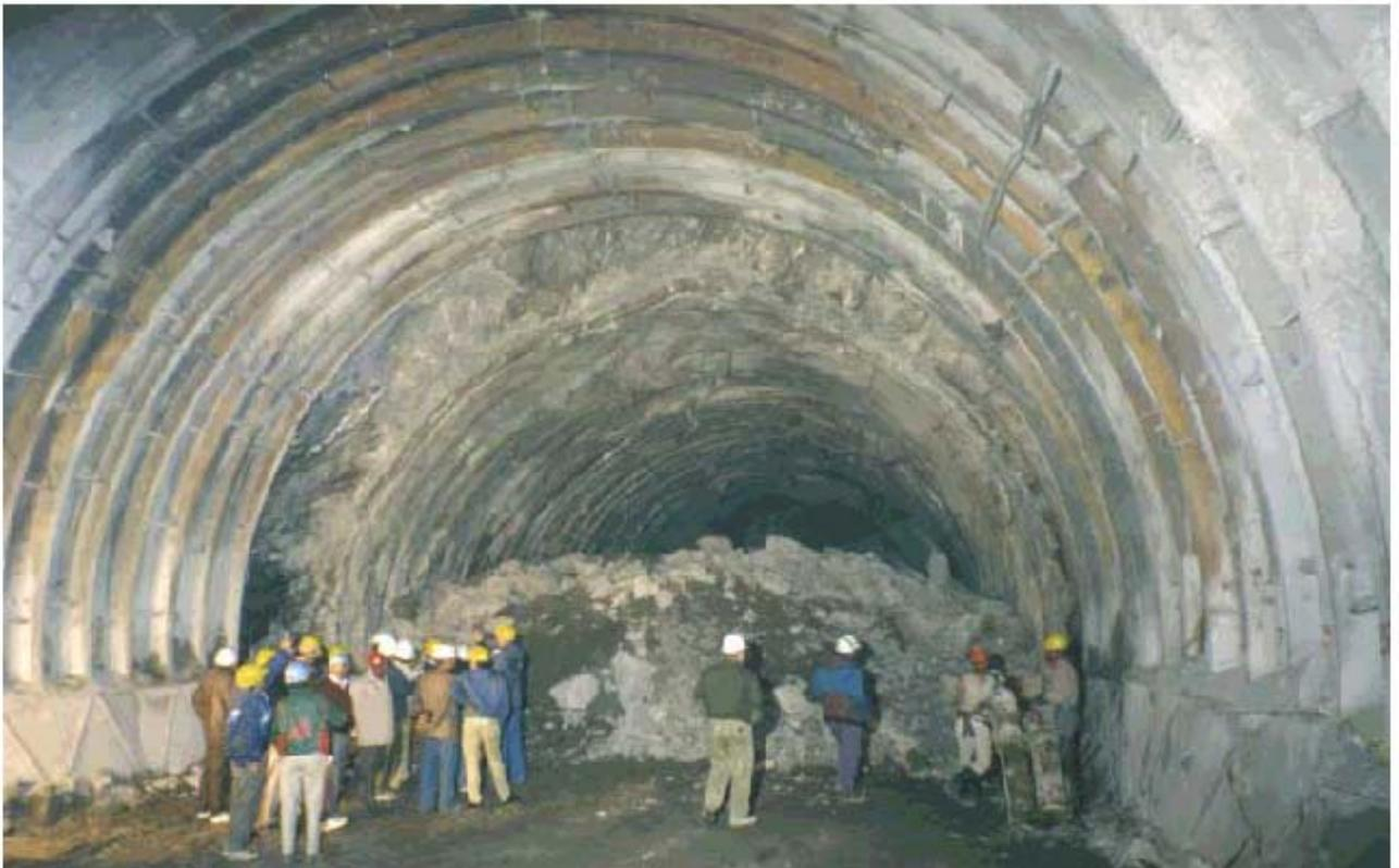
Figure 7: Large convergence in the Nathpa Jhakri headrace tunnel top heading due to the influence of the Daj Khad shear zone.
